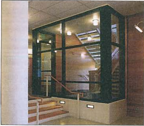
PROJECT: Evergreen Aviation & Space Museum, McMinnville, Ore. PRODUCT: Technical Glass Products' Pilkington Pyrostop Transparent Wall Panels USE: TGP applied at the home of the world-famous Spruce Goose flying boat airplane to create a fire-resistive stairwell enclosure CONTACT: fireglass.com, Circle 522 PHOTO: Pete Eckert
