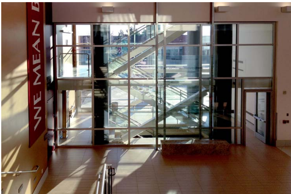
SuperLite II-XL in GPX Framing was used in this 2-hour stairwell to enable views to the outdoors and allow natural daylight to penetrate further in the building. (Project: David Eccles School of Business at the University of Utah. Architect: MHTN Architects. Glazier: Mollerup Glass)
