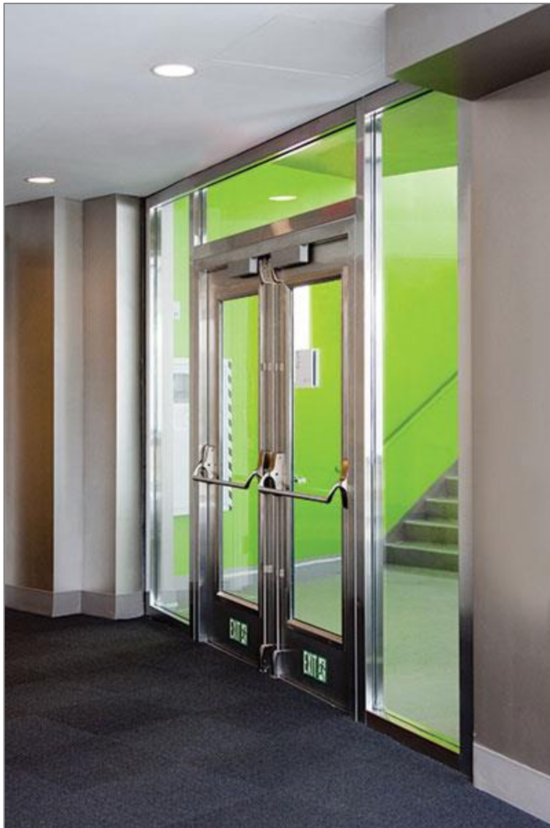
For this 2-hour stairwell, SuperLite II-XL 90 is used to exceed 100 sq. in. in the door vision panels while SuperLite II-XL 120 in Stainless Steel GPX Framing is used for the sidelites and transoms. Architect: KPF. Glazier: RG Creation. Project: CUNY School of Law in Long Island City, NY.
