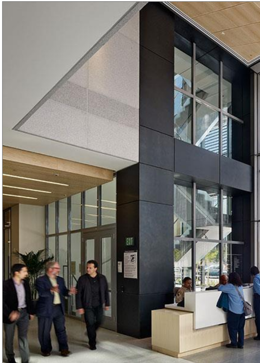
SuperLite II-XL 120 in GPX Framing is used on all 14-floors of the LEED Platinum-certified San Francisco Public Utilities Commission Building. This transparent 2-hour stairwell help bring daylight deeper into the building. Architect: KMD. Glazier: Progress Glass.
