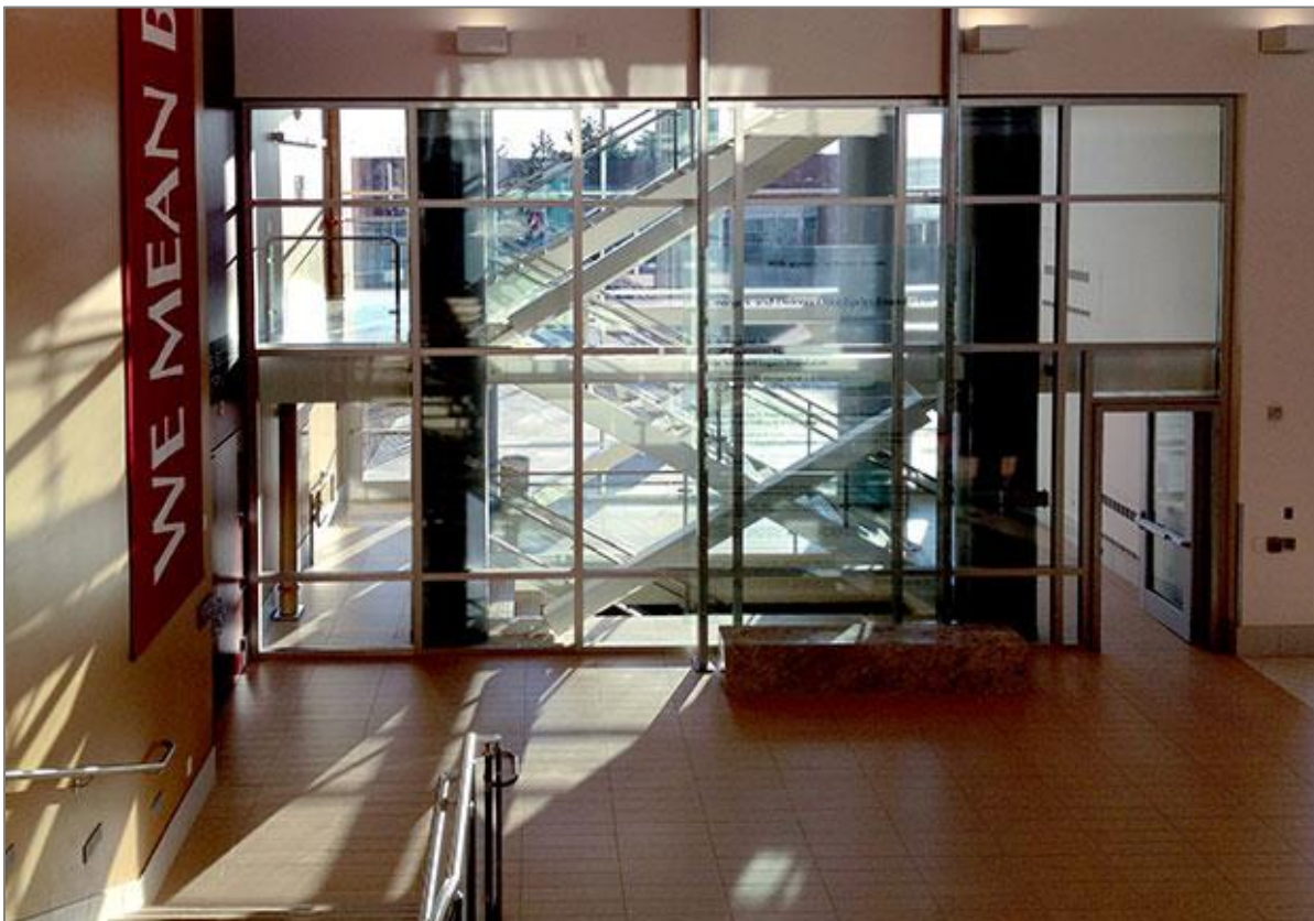
SuperLite II-XL 120 in GPX Framing add daylight and transparency to this 2-hour stairwell. Architect: MHTN Architects. Glazier: Mollerup Glass. Project: David Eccles School of Business at the University of UT in Salt Lake City, UT.
