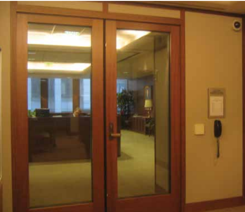
Ballistic pair doors with cherry wood veneer at a private office in San Francisco, Calif.
