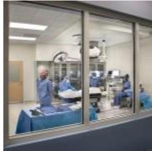
**Central Carolina Technical College, Sumter, South Carolina.** SuperLite II-XL 60 in GPX framing was used in the openings in this 1-hour exit corridor because the total glass area exceeded 25% of the wall. The college needed extensive openings for observation.
