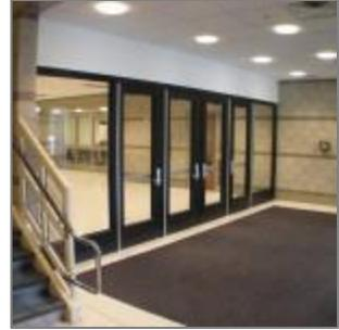
**Michigan Technical Education Center, Kalamazoo, Michigan.** To meet the code requirements of this 1-hour fire barrier, SAFTI FIRST supplied SuperLite II-XL 60 in GPX door framing and SuperLite II-XL 60 in GPX wall framing. Because the vision areas in the doors exceed 100 square inches and the architect wanted to incorporate glass in this application, fire-resistive ASTM E-119 rated SuperLite II-XL and GPX framing were used.
