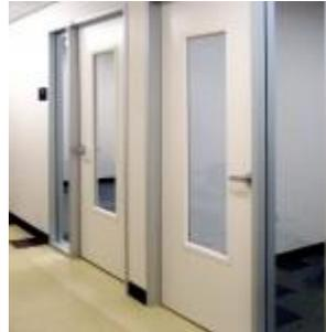
**National Center for International Schools (NCIS), San Francisco, California.** This 1-hour exit corridor used SuperLite I in the 20-minute rated doors, and Superlite I-XL in the 45-minute rated sidelites. NCIS selected SuperLite I-XL because it offers partial protection from radiant heat transfer and is more cost-effective when compared to filmed or laminated ceramic.
