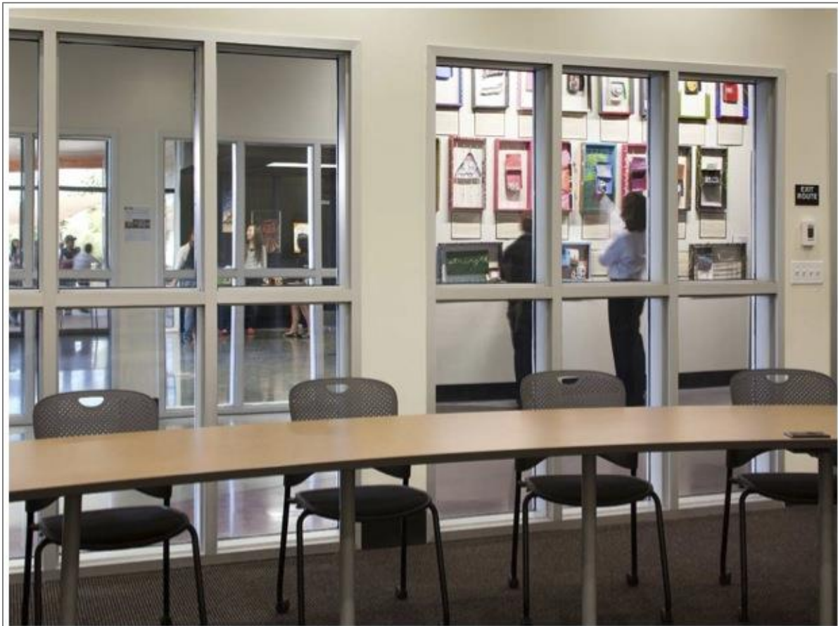
High Tech Middle School in Chula Vista, California, chose SuperLite II-XL 45 in HM Framing by SAFTIFIRST for the fire protective openings in this 1 hour corridor. SuperLite II-XL 45 also has an STC 40 rating providing sound attenuation benefits to go along with clear views and fire protection.
