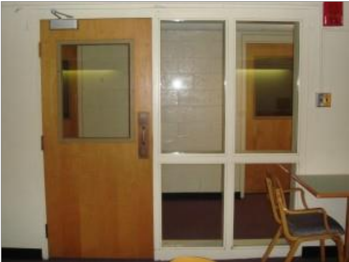
Middlebury College replaced unsafe wired glass in and around this dormitory door with SuperLite I (vision panel) and SuperLite II-XL (sidelites)
