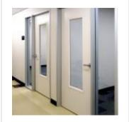
Central Carolina Technical College, Sumter, South Carolina. SuperLite II-XL 60 in GPX framing was used in the openings in this 1-hour exit corridor because the total glass area exceeded 25% of the wall. The college needed extensive openings for observation.
