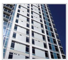
The SuperLite II-XL 45 IGU are used as opening protectives for the part of the building that is adjacent to the lot line. The glazing is marked OH-45 and is subject to size limitations.
