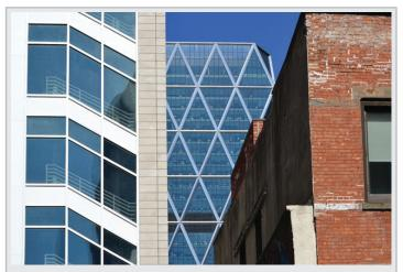
Because the building on the left uses a significant amount of glazing while in close proximity to the adjacent brick building on the right, a fire-resistance-rated wall assembly using SuperLite II-XL 60 in GPX Curtain Wall framing was used meet code requirements. The glazing is marked W-60 to signify that it meets ASTM E-119.
