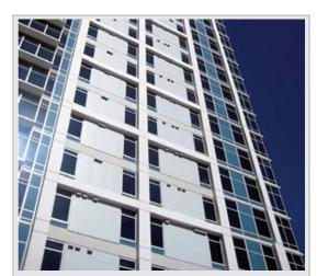
The SuperLite II-XL 45 IGU are used as opening protectives for the part of the building that is adjacent to the lot line. The glazing is marked OH-45 and is subject to size limitations.
