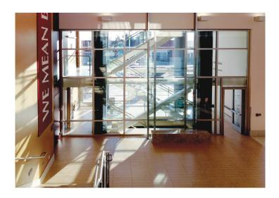
This two hour wall is an example of how GPX Architectural Series with SuperLite II-XL 120 glazing enhances interior spaces with elegant transparency and natural daylight during everyday use, and protects building occupants from the potentially devastating effects of radiant heat by ensuring safe egress during a fire.
