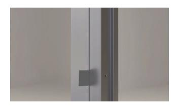
Once the door frame is level, square and plumb, drill through the top mounting hole if needed, to set first mounting screw. Use the provided anchors.
