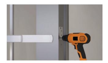
Once the door is hung, check the swing to make sure the gaps are consistent with the shop drawings and within tolerance. Also check to make sure the door is opening and closing smoothly.
