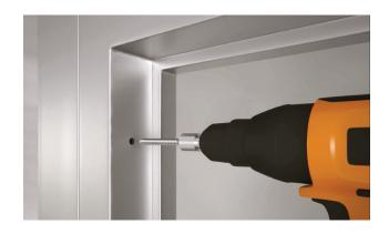
Check for square by measuring from the top left corner to the bottom right corner, then the top right corner to the bottom left corner. Continue the door frame installation using the provided anchors. Measure periodically, making sure it is level, square and plumb. Make adjustments if necessary.
