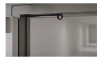
Check the swing again. Adjust the closer so that the required door opening force is satisfied (30 pounds of force to set in motion, 15 pounds of force to complete the swing). Reference the door's installation instructions when adjusting the swing and latch speeds. Adjust the strikes if necessary.
