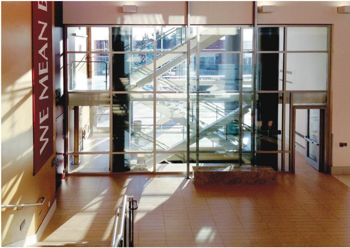
This two hour wall is an example of how GPX Framing with SuperLite II-XL 120 glazing enhances interior spaces with elegant transparency and natural daylight during everyday use, and protects building occupants from the potentially devastating effects of radiant heat by ensuring safe egress during a fire.
