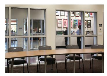
For this 1-hour corridor, the design team chose SuperLite II-XL 45 for its superior optical clarity, CPSC Cat. II impact safety ratings, high STC ratings and full radiant heat protection at a fraction of the cost of tinted filmed or laminated ceramic used in the same application.
