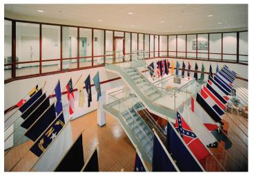
SuperLite II-XL 60 and GPX Framing were used to create a transparent wall system that seamlessly combines vision and light with maximum fire protection. This fire rated system also provides smooth, angular transitions along the corners to achieve the designer's intent to have a beautiful viewing area that highlights the building's focal point.
