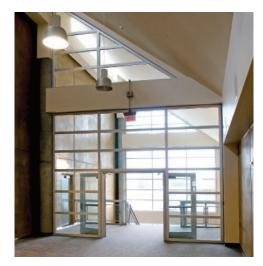
Fire resistive GPX Doors and Framing with SuperLite II-XL glazing provide transparency to this two-hour wall; enhancing the sense of openness by maximizing natural light in interior spaces, with the added benefits of safe egress and personal security.
