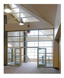
Fire resistive SuperLite II-XL in GPX Architectural Series Framing (including Doors) provides transparency to this two-hour wall; enhancing the sense of openness by maximizing natural light in interior spaces, with the added benefits of safe egress and personal security.
