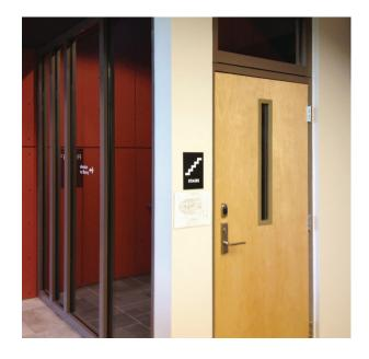
SuperLite X-45/60/90 is listed and labeled by Intertek and Underwriters Laboratories, nationally recognized testing laboratories approved by OSHA.
