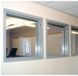
This San Francisco school selected SuperLite I-XL to replace unsafe traditional wired glass, in order to benefit from its partial radiant heat protection and high impact resistance. The use of SuperLite I-XL ensures that students can safely pass through the corridors on a normal daily basis and during an emergency such as an earthquake or fire.
