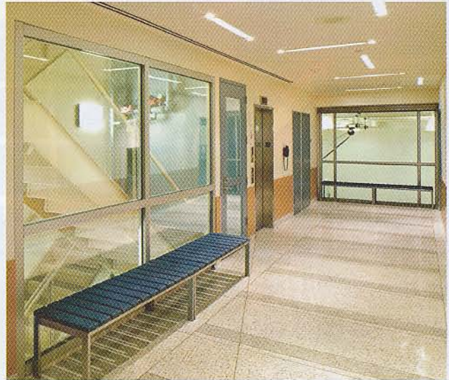
Platt Byard Dovell White Architects specified 120-minute fire-resistive glazing for the Reece School in New York to enhance the building's transparency while still protecting the occupants.
