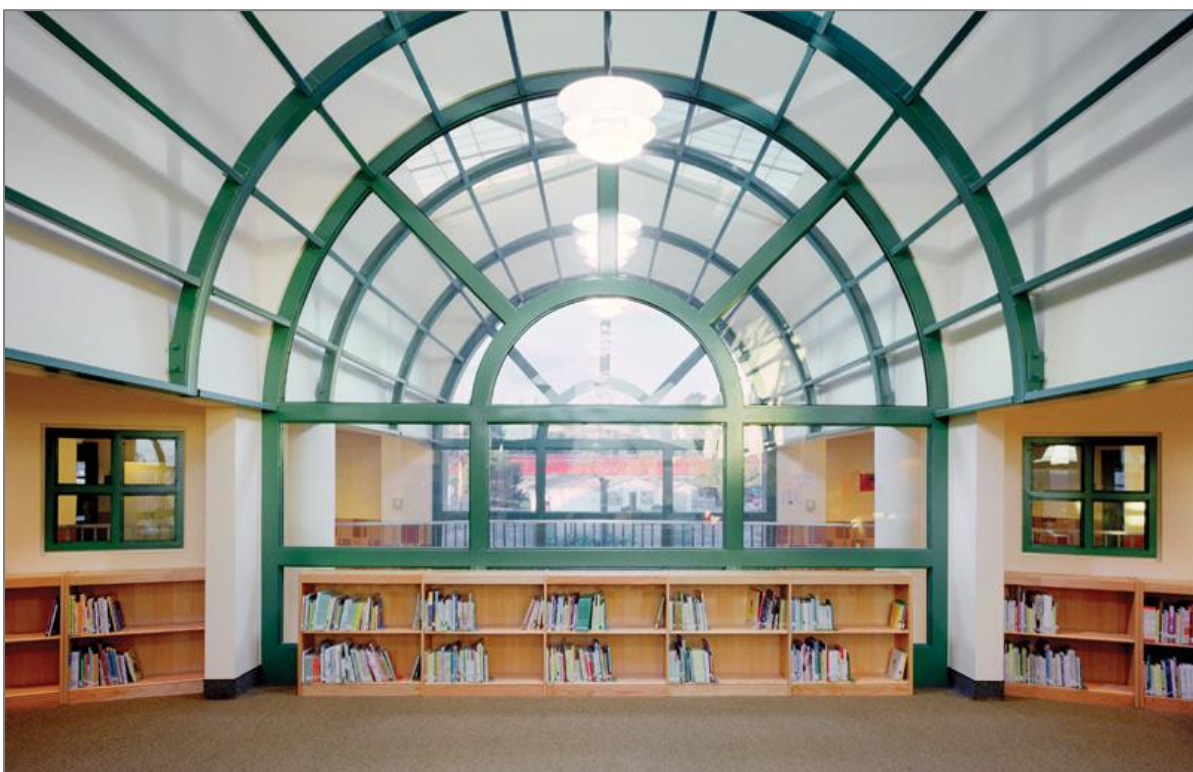
Fire rated glazing in the library at Sunset Elementary in San Ysidro CA pulls in day light.
