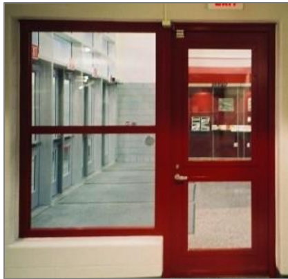
2-hour exit passageway, Troy HS, Ohio
